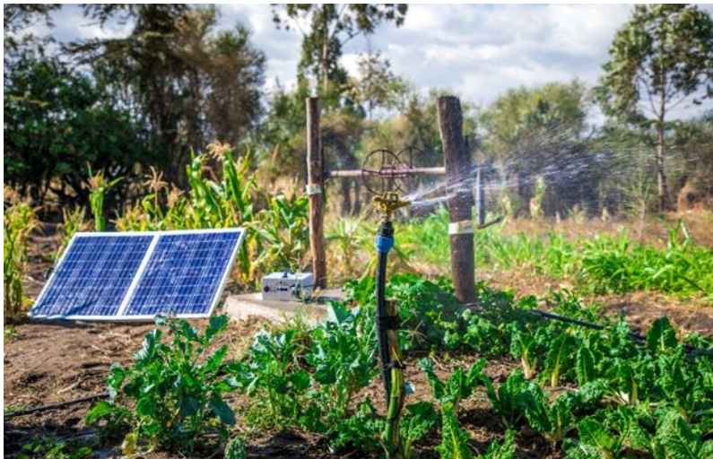
Solar Pumping in Operation
