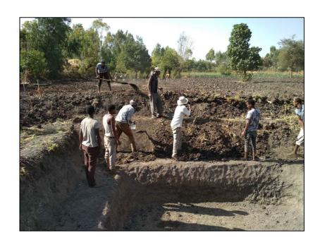
Continue to remove the steps and to straighten the slope between rectangle 3 and 4. Work your way down from 3 to 4. All removed soil is to be added to the embankments.
