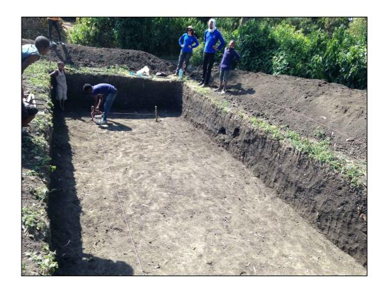
After all dimensions are double checked, start digging, The second excavation, 1 meter depth.
